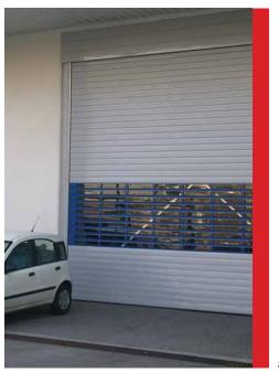
PROFILE A: ALUMINUM DIMENSION: 140mm THICKNESS: 0,6mm
