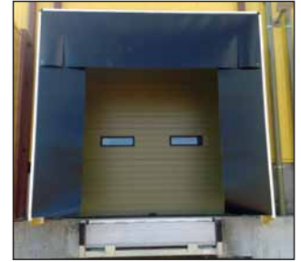
Accordion shutter embedded in the factory wall with encased loading ramp.
